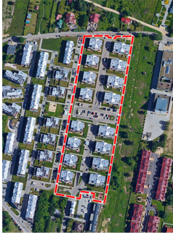
Figure 1. The land use and boundaries of the housing estate area included in the analysis [77].
